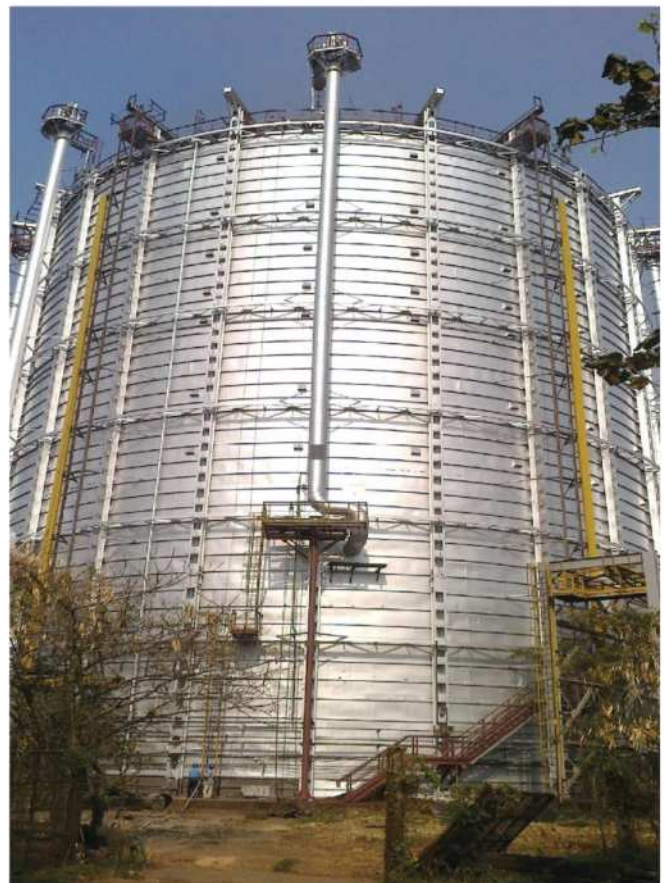
DISMANTLING & EPC OF BOF GAS HOLDER AT SAIL, DURGAPUR
