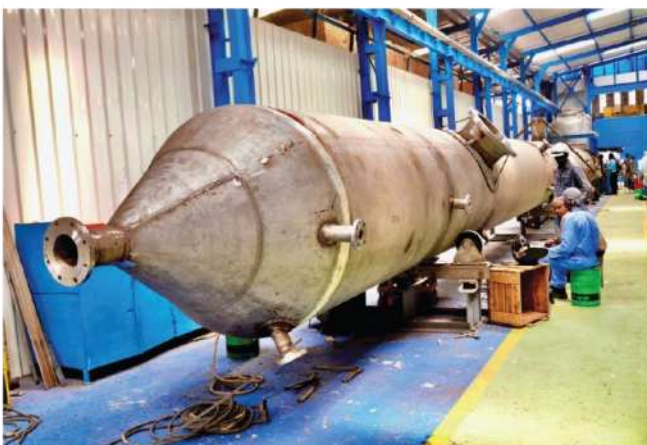
DE-NITRATION PLANT PROJECT FOR HEAVY WATER BOARD
