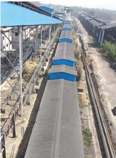
COAL HANDLING PLANT AT NBPPL, UNCHAHAR
