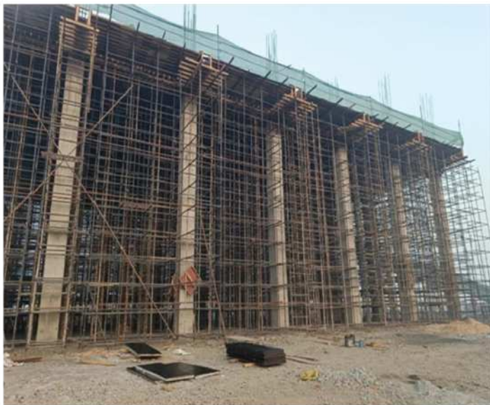
UREA HANDLING & BAGGING PACKAGE AT TFL, TALCHER
