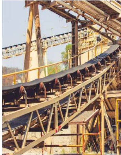
COAL HANDLING PLANT AT NORTH KARANPURA
