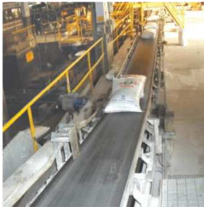
EPC FOR BAGGING PLANT EXPANSION AT TCL, BABRALA
