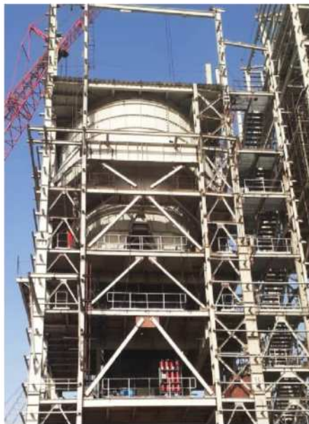
COMPLETE MECHANIZED COAL HANDLING SYSTEM WITH 10000 TONS RCC OVERGROUND BUNKER WITH RAPID LOADING SYSTEM FOR NTPC - PAKRI BARWADIH MINES
