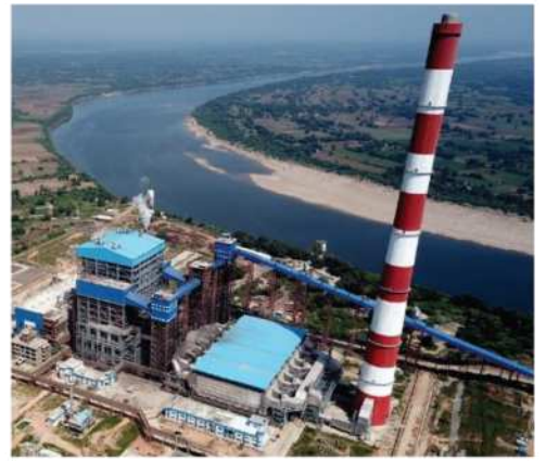
CHP AT BHEL WANAKBORI (1X800MW) EXTENSION TPS UNIT # 8 (GSECL)
