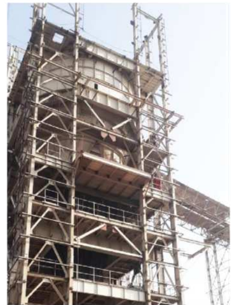
COMPLETE MECHANIZED COAL HANDLING SYSTEM WITH 10000 TONS RCC OVERGROUND BUNKER WITH RAPID LOADING SYSTEM FOR NTPC - PAKRI BARWADIH MINES
